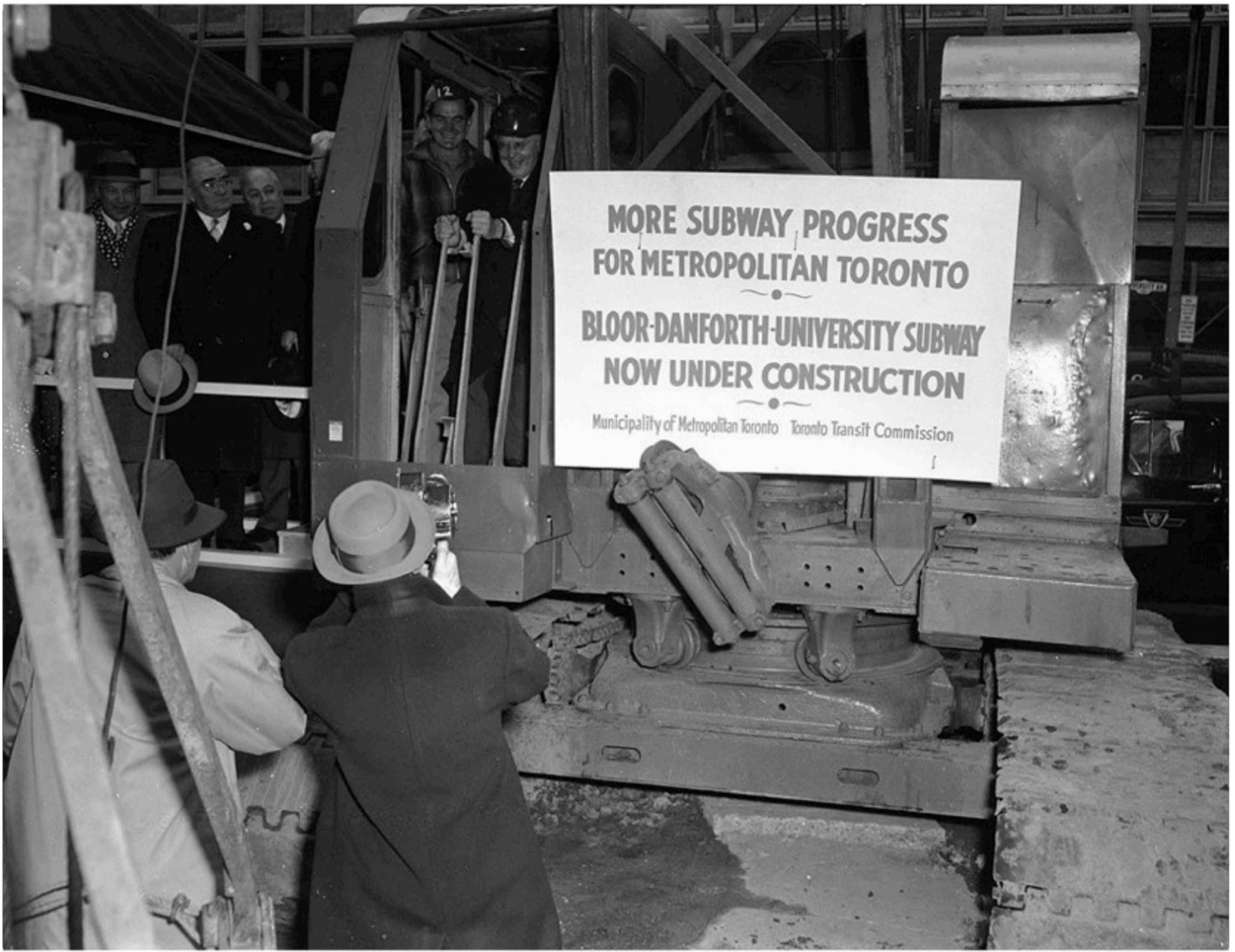
Opening of Construction, 1959 City of Toronto Archives, Fonds 1567, Series 648, Item 17
