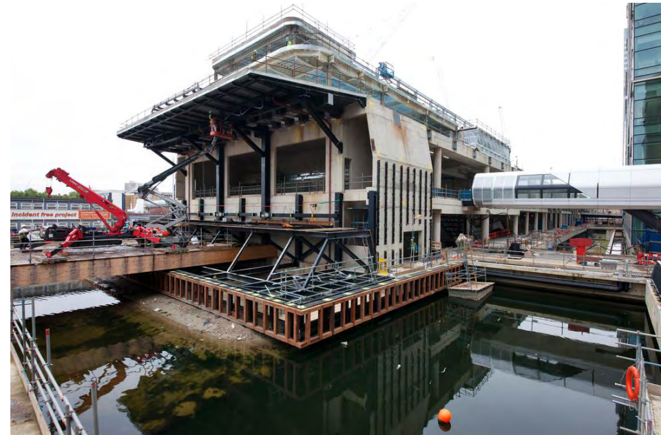
Station Construction September 2013
